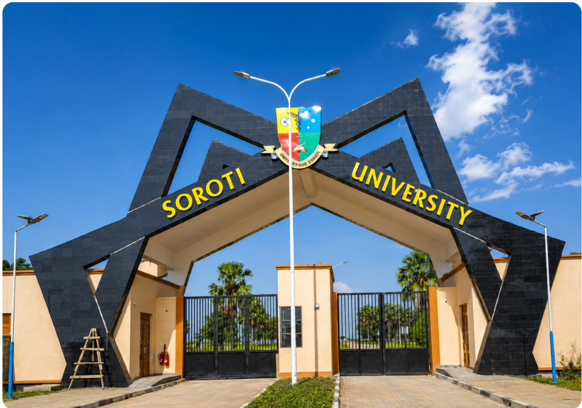
SOROTI UNIVERSITY MAIN GATE
